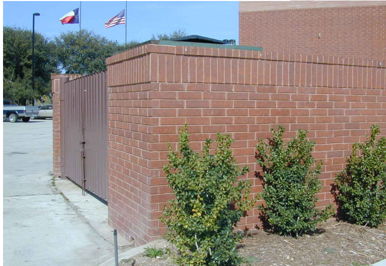
Figure 4.07.3. Example of Refuse Area Screening
