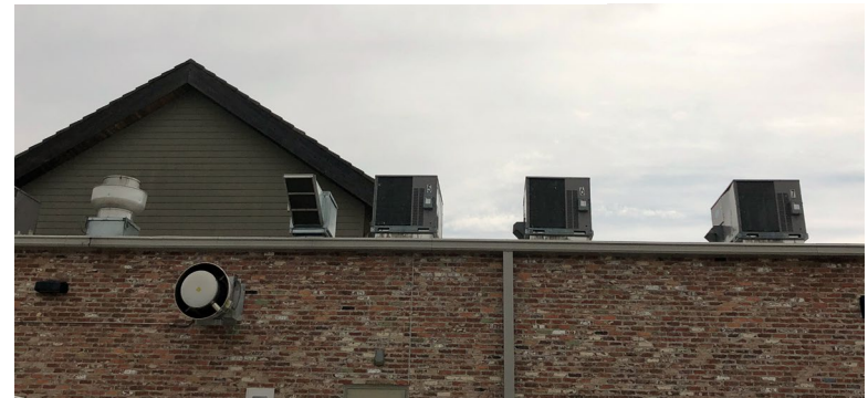
Figure 4.07.4. Example of Unscreened Rooftop
